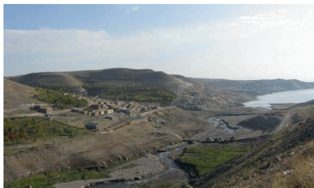
Fig. 1 Sediments behind the Alavian Dam at the exit of the Ashan drainage basin.
